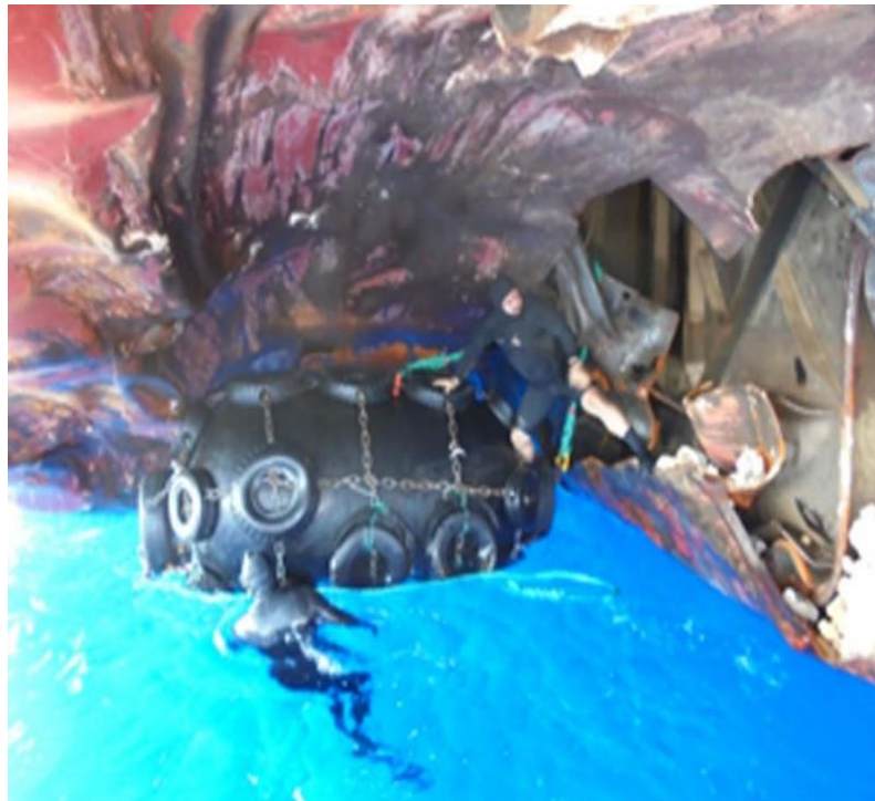
Figure 22. The yokohama fender secured on Ince Inebolu bulbous bow (source Tsavliris Salvage).
