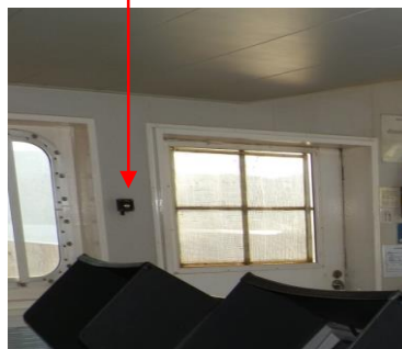
Figure 34. The Remote Reset Unit on port bulkhead.
